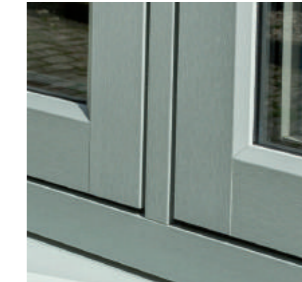
TIMBERWELD JOINT
